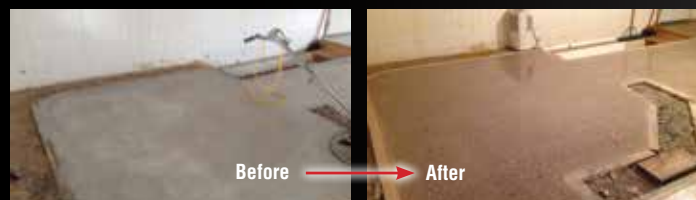
Concrete Polishing
