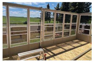
This customer wanted a covered deck edition to go with their sunroom. After all pieces are in place for the sunroom, they move to completing the roof over the deck and adding a support to ensure stability. Gutters and fascia are installed once the roofing system is finished. To complete the project, they will use Sunspace AlumaDeck and railings on the covered deck and finish with stairs.
